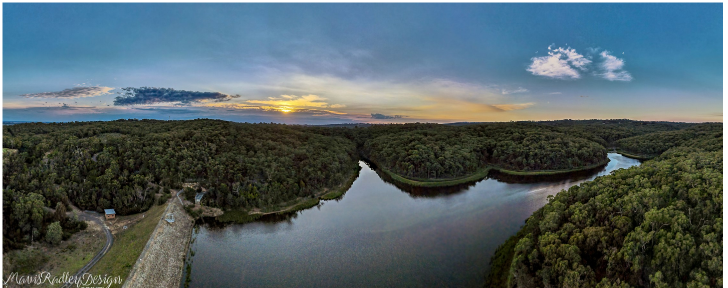
Beaconsfield Reservoir looking west showing existing dam wall prior to lowering of the water level commencing.
