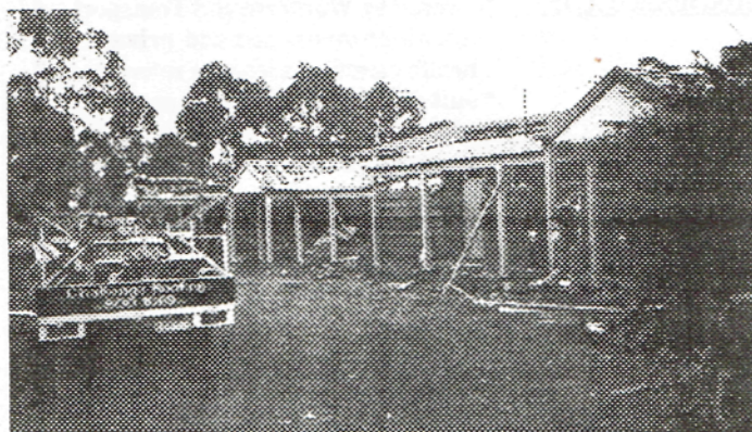
Melaleuca Lodge as renovations near completion.
