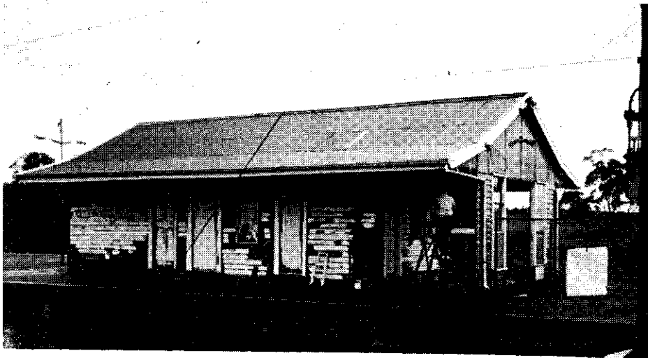
(Above) Beaconsfield Railway Station with the "Stop Tar" applied.
